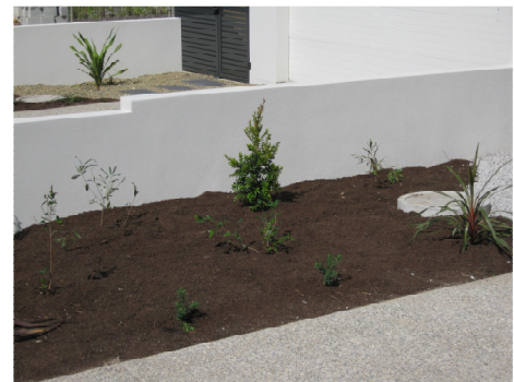
6,200Lt under ground tanks Sunshine Cove located under the driveway and garden area
